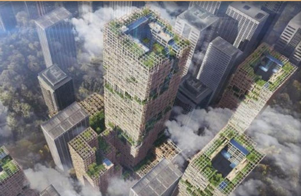
A Japanese company is set to build a skyscraper made of 90% wood in Tokyo, which will make it the world's tallest wooden skyscraper upon completion. The wooden high-rise, named "W350", will be a "braced tube structure" at 350 meters (1,150 ft) tall and 70 stories. To construct it, 180,000 cubic meters of wood will be combined with the other 10% of the building's makeup—steel.
