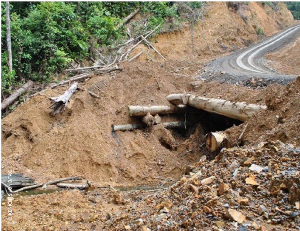
*A logging road with an improperly constructed stream crossing*
